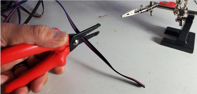
2. Separate  $\frac{1}{2}$ " of wires from both sides of RGB cable
